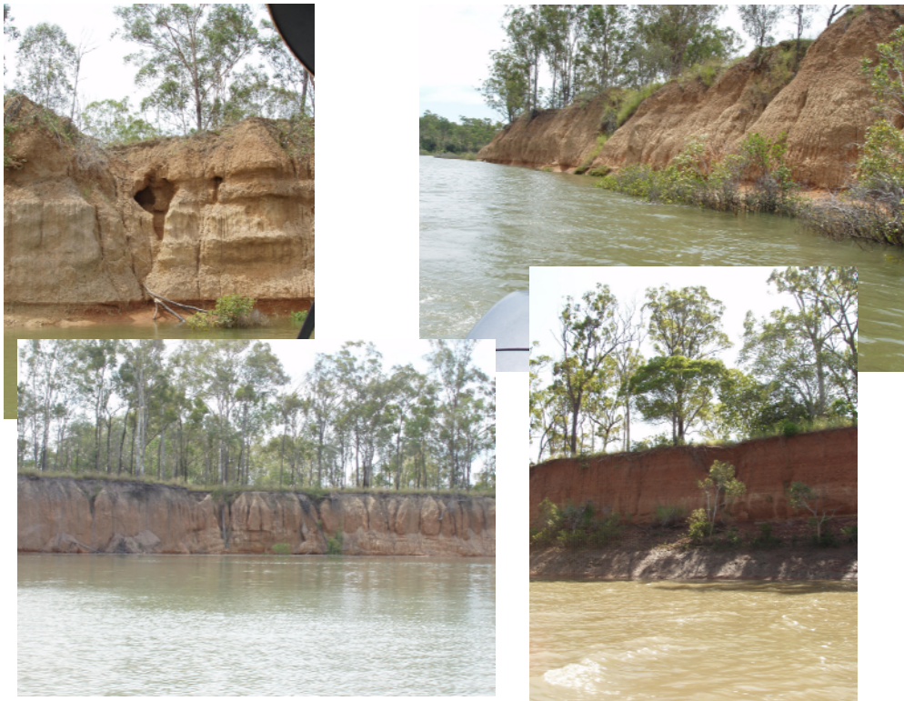
Photographs along Calliope River showing evidence of bank erosion
